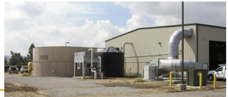
RP-5 Manure Digester Building
