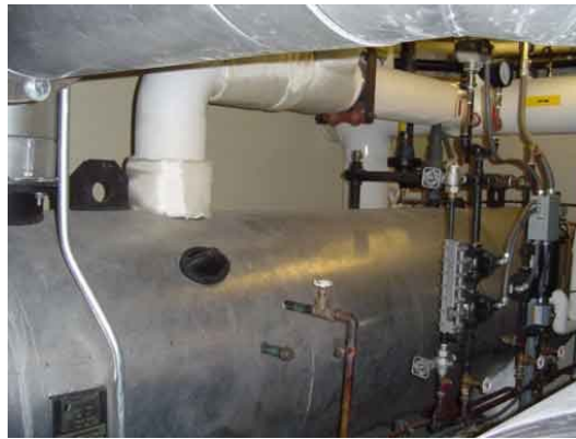
Heat Recovery Steam Generator
