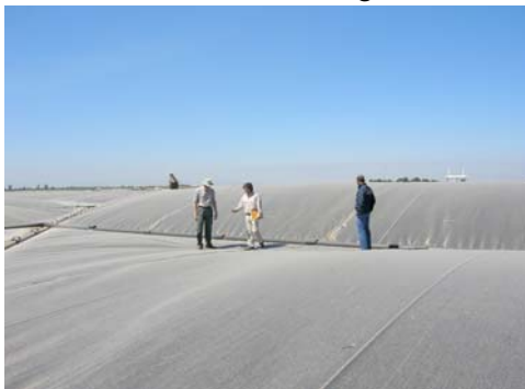
Picture below: the 7 acre digester cover
