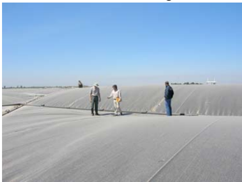
Picture below: the 7 acre digester cover
