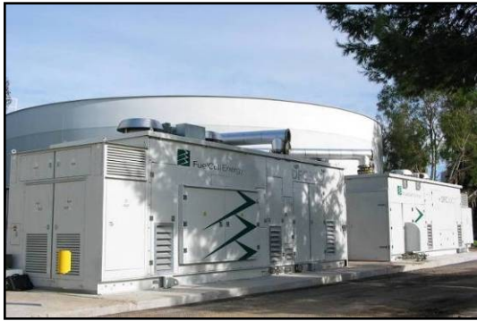
Wastewater Treatment, Santa Barbara, CA
